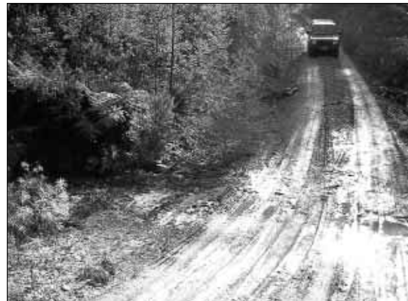
Runoff accumulates quickly on compacted road surfaces even during light to moderate rainfall
