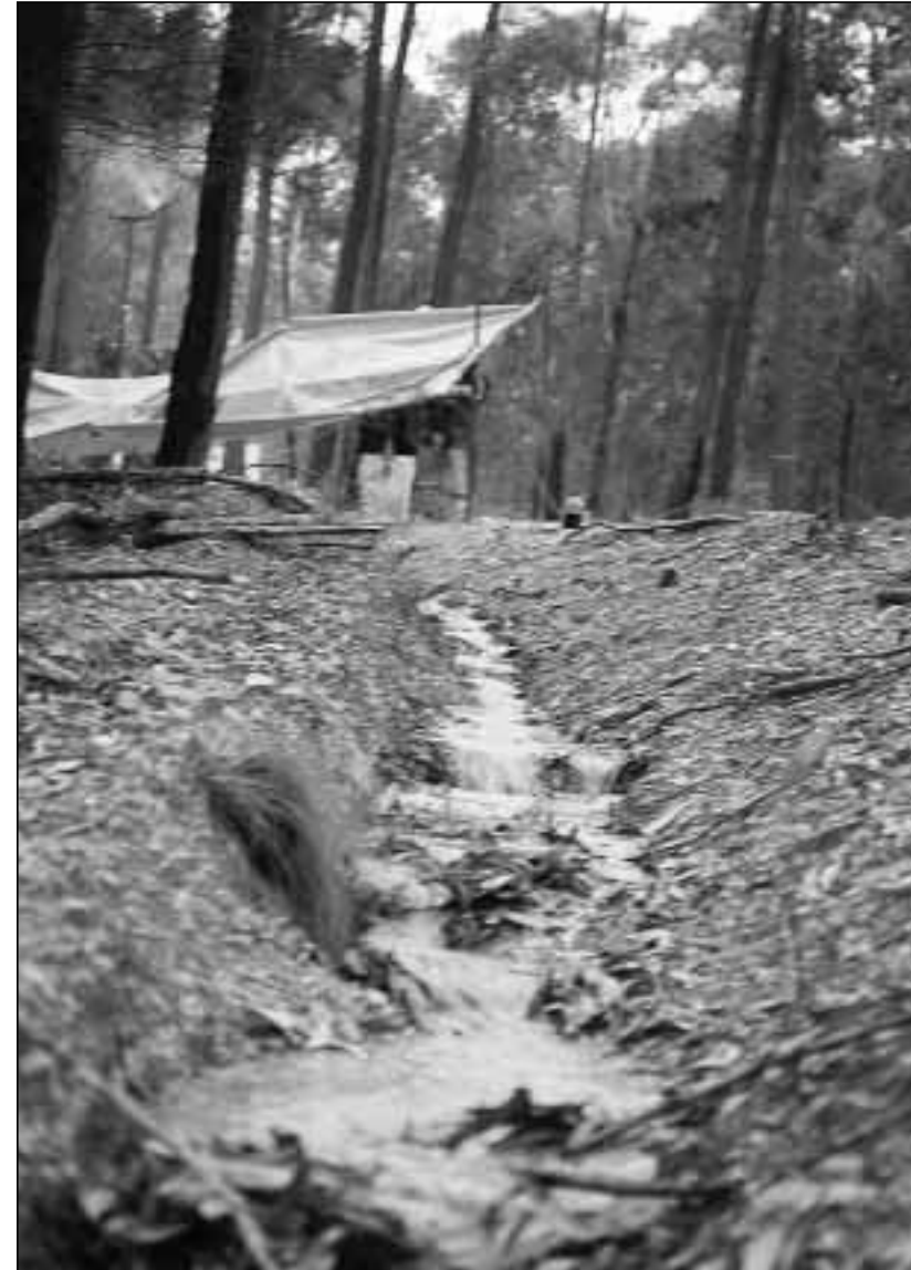
Water discharging from mitre drain and travelling downslope across vegetated surface, where flow quickly spreads and disperses across the hillslope
