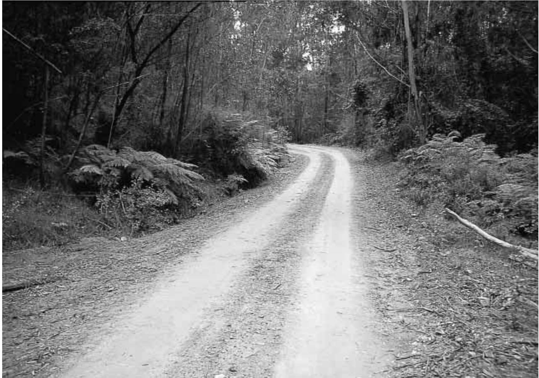
Appropriate siting of unsealed forest roads is critical in reducing sediment and nutrient loads to streams.
